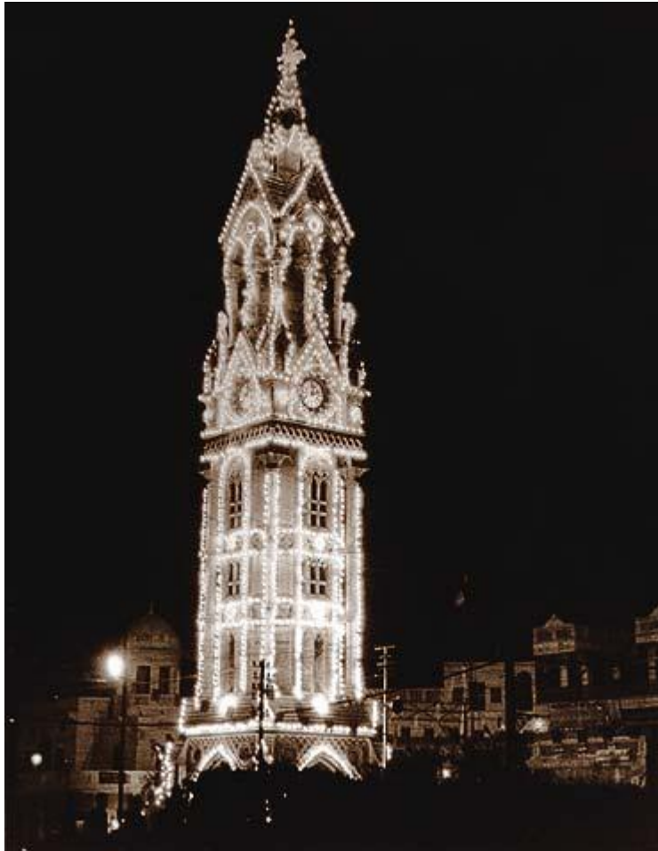
Midnight Aug 14, 1947 The Ghanta Ghar illuminated. It collapsed a few years later.
